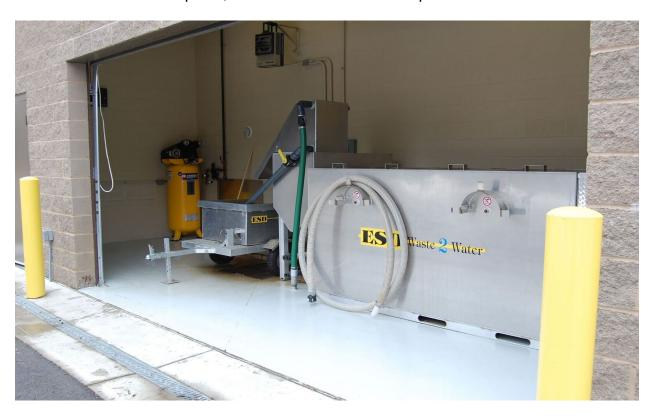
Figure 33. Wash equipment over a concrete or asphalt pad that allows the water to be collected. Photo credit: Jason Mahl.
