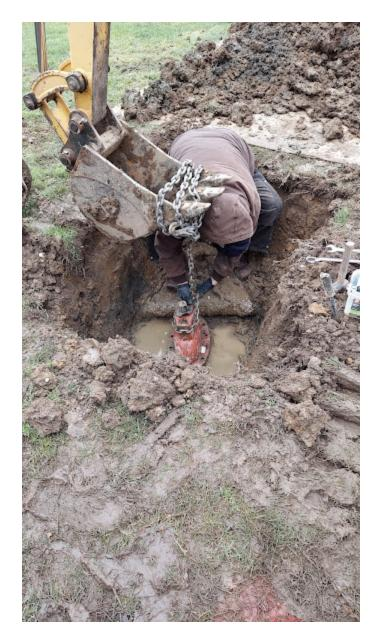
Figure 10. Valves should be repaired as necessary so that proper maintenance of the irrigation system can be performed.
