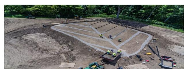
Figure 3. When constructing drainage systems, pay close attention to engineering details such as subsoil preparation, the placement of gravel, slopes, and backfilling. Photo credit: Jason Mahl.
