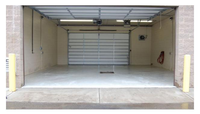
Figure 4. Construct floors of seamless metal or concrete sealed with a chemical-resistant paint. Photo credit: Jason Mahl.
