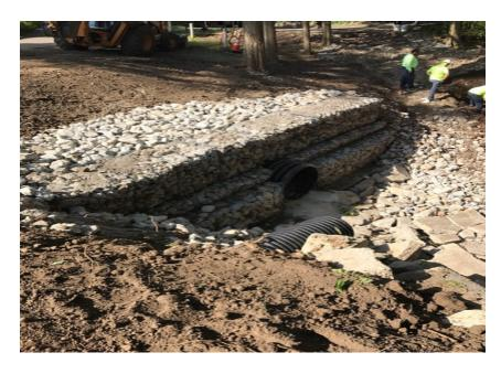
Figure 14. Use detention basins/catchments and water quality practices to buffer flooding and excessive runoff that may contain sediment. Photo credit: Ryan D'Autremont.
